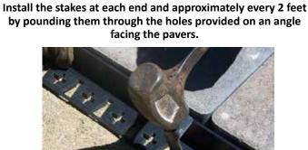
This unique and versatile "L" shape paver restraint is comes in six foot (6') lengths. It can be used as a rigid straight piece OR easily converted to use with curves by use of a hand pruner. Use with standard paving stones and patio stones. May also be used as a landscape border around a bedding area with stone/mulch. Extra heavy duty poly anchor stakes are included in order to ensure that you have more than enough to get the job done right
