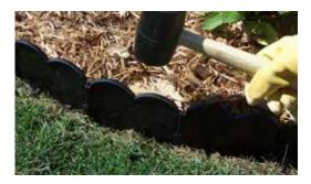
Insert next piece into the hinged connection point sliding straight down. When the new piece is to the point of touching the ground, pound it down to grade level point like previous piece. Continue this step until design is complete.
